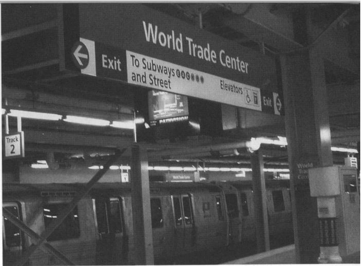
A simple blue and white sign dramatically proclaims that PATH trains have returned to their Lower Manhattan terminal.
